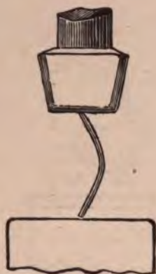
Fig. 5—Bending Still Further by means of a Steam Hammer.
