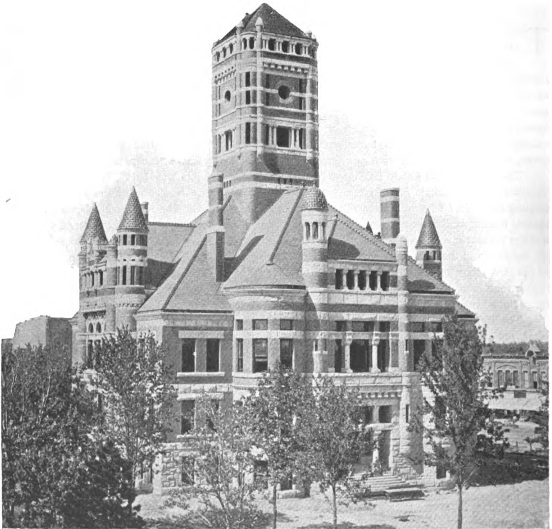
Williams County Court House, Bryan, Ohio.
