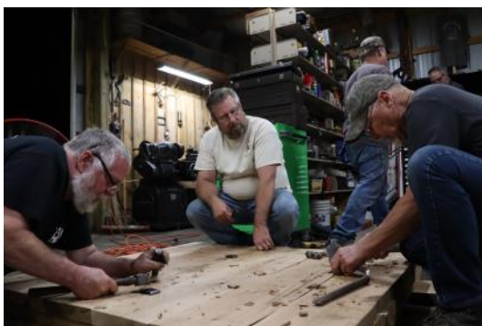
Chiseling out for the bolts to go through the bottom
