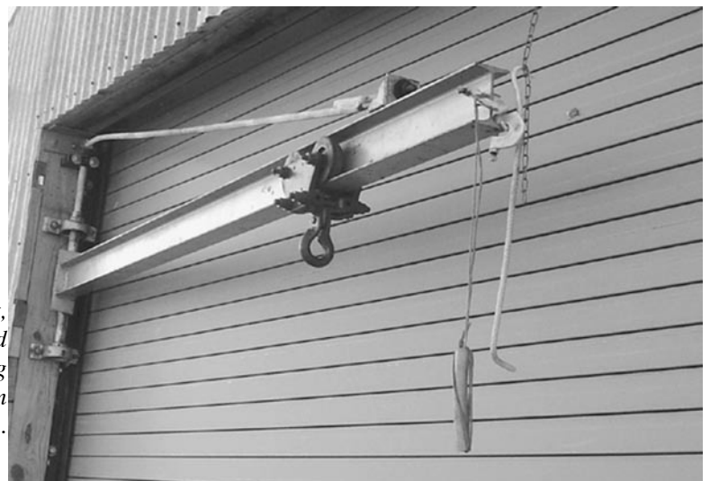
Right, Finished working crane in place.
