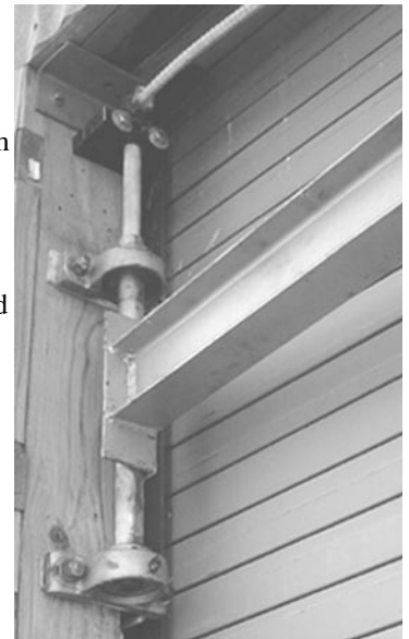
Close up of bearing setup
