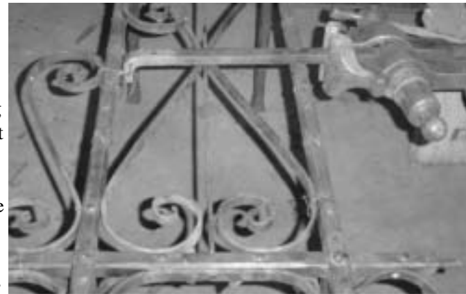
Using a bucking bar to back up the rivets.
