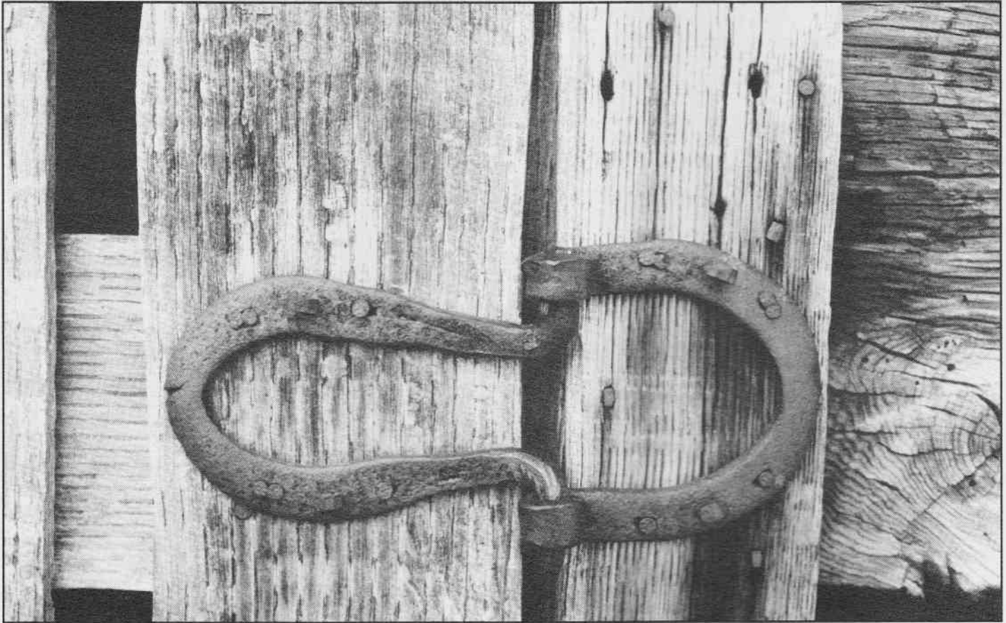
This unique hinge was on a door of an outbuilding that is part of the Great Smoky Mountains National Park visitor's center in North Carolina. The graceful lines of true folk art are apparent though the maker was more concerned with function than form. Photo by Jim McCarty.
