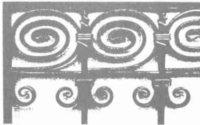
Detail of dining room door grille Brad Silberberg Bradley Metal Design, Inc.
